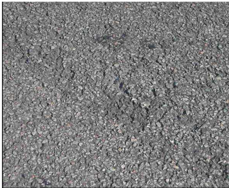
Figure C6 Ravelling and fretting
