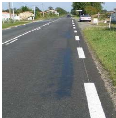
Figure C10 bleeding or fatting up of UTLAC (loss of macro-texture)
